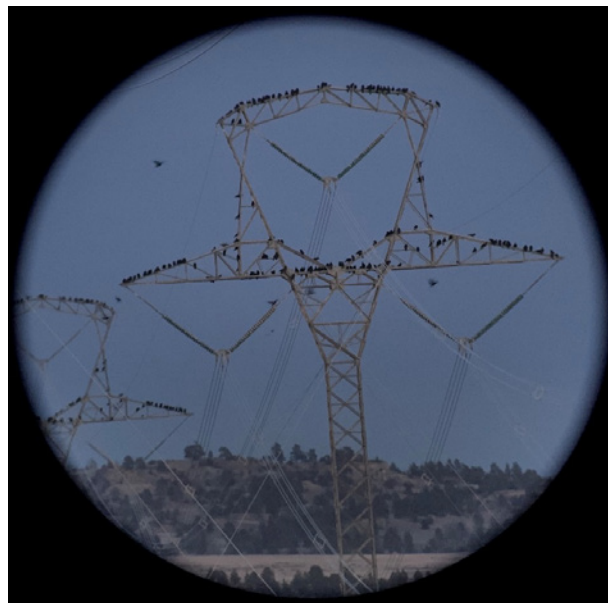
Figure 4-4. Ravens Roosting on a 500 kV Tower
